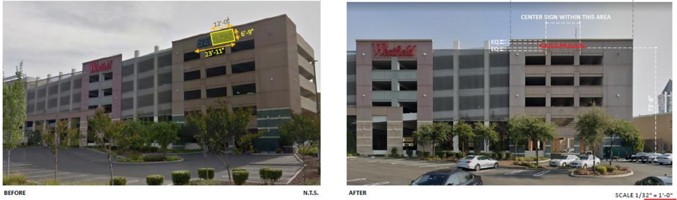
Figure 5: Parking Garage Sign (Before and After)
